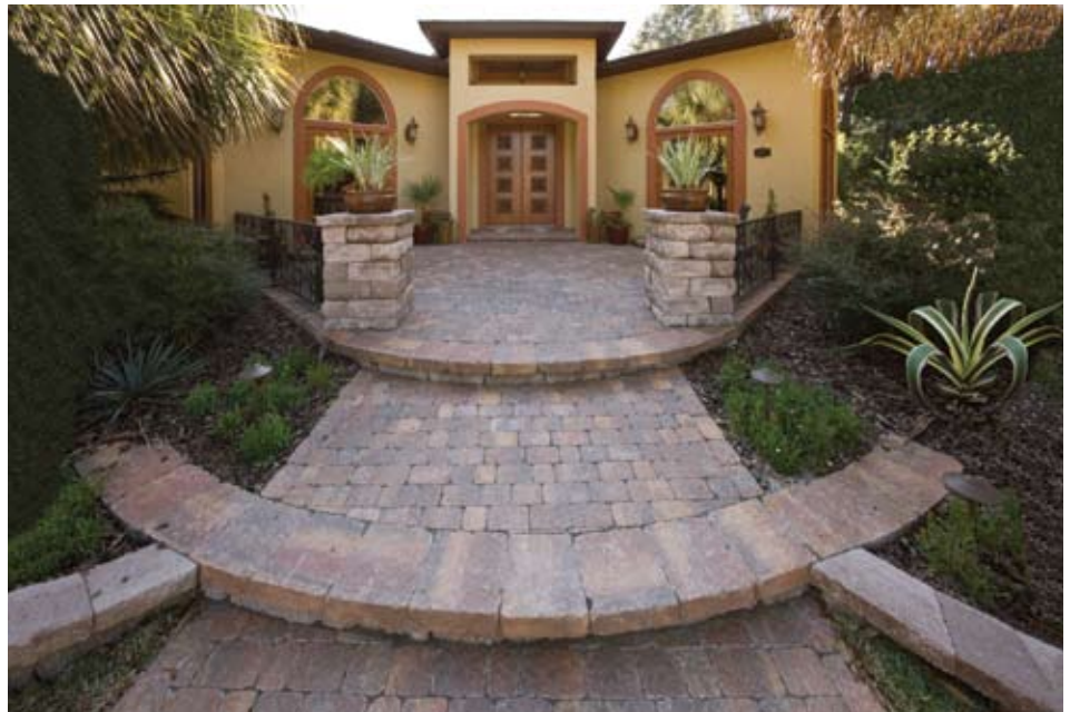
The remodeling work on this home included creation of this extremely unique front entry.
